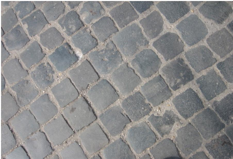
Figure 49 – Pavement of the tunnel: cobblestones (Sampietrini)
