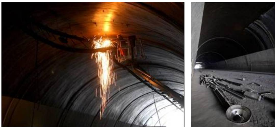
Figure 6 – Removal of existing lighting system
