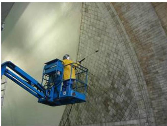
Figure 7 – Washing and cleaning of the vault
