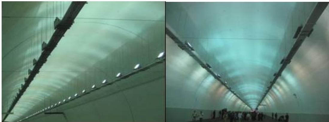
Figure 13 – Position and types of lamp
