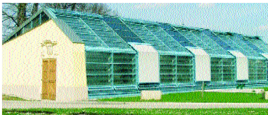
Building of the technology incubator
