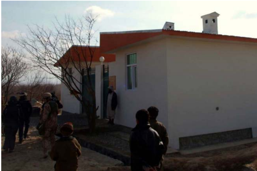
Milk collection centre – outside the new building
