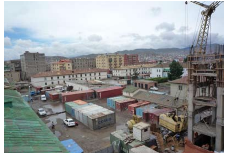
The old micro district will be leveled and new apartments built
