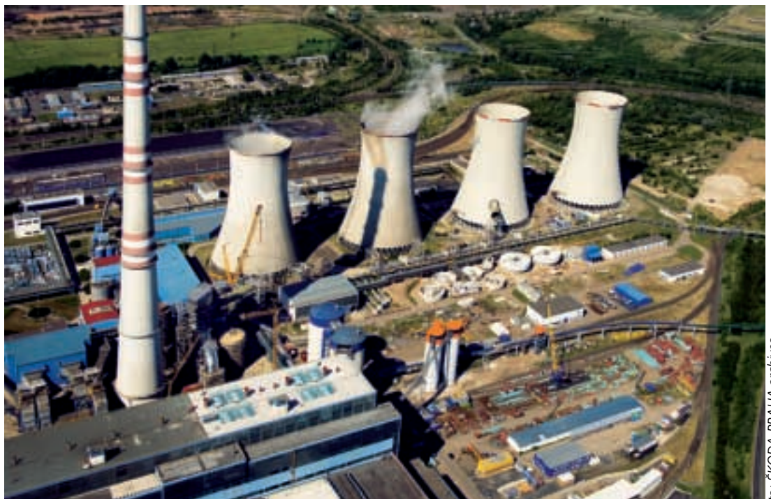
Tušimice thermal power plant
