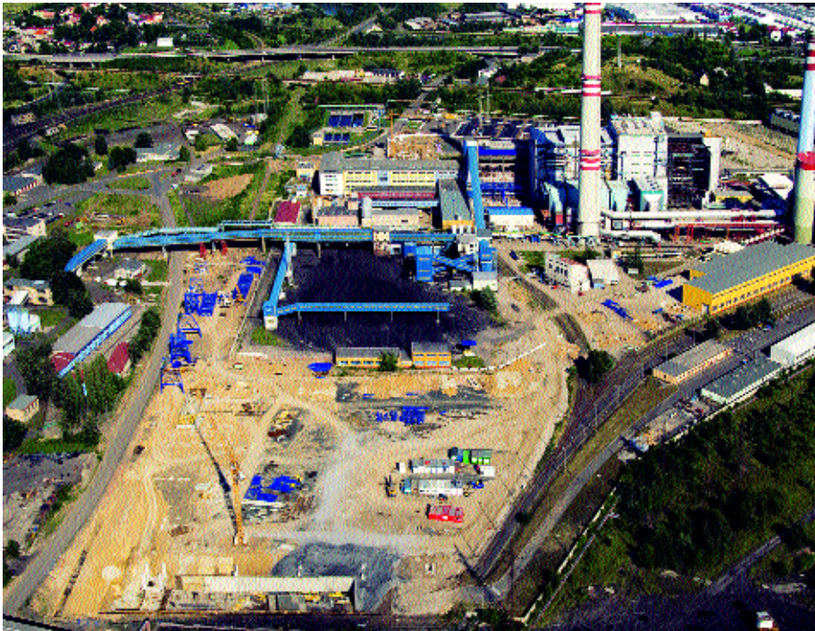
Ledvice thermal power plant
