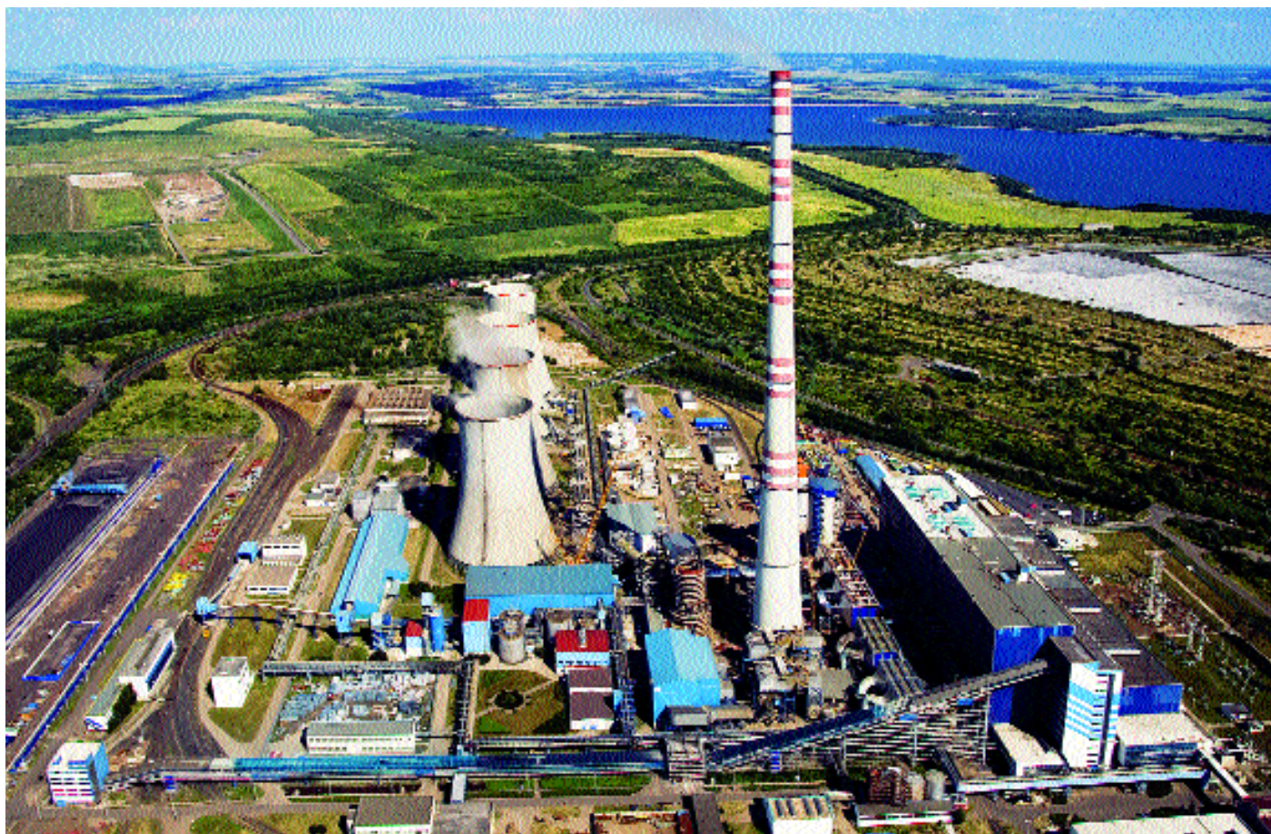
Tušimice thermal power plant
