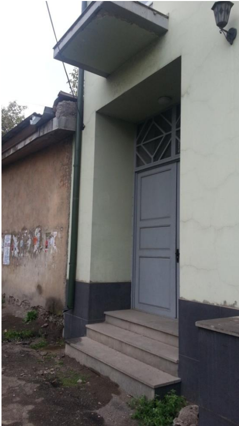
The main entrance to the Akhalsikhe rural service centre.
