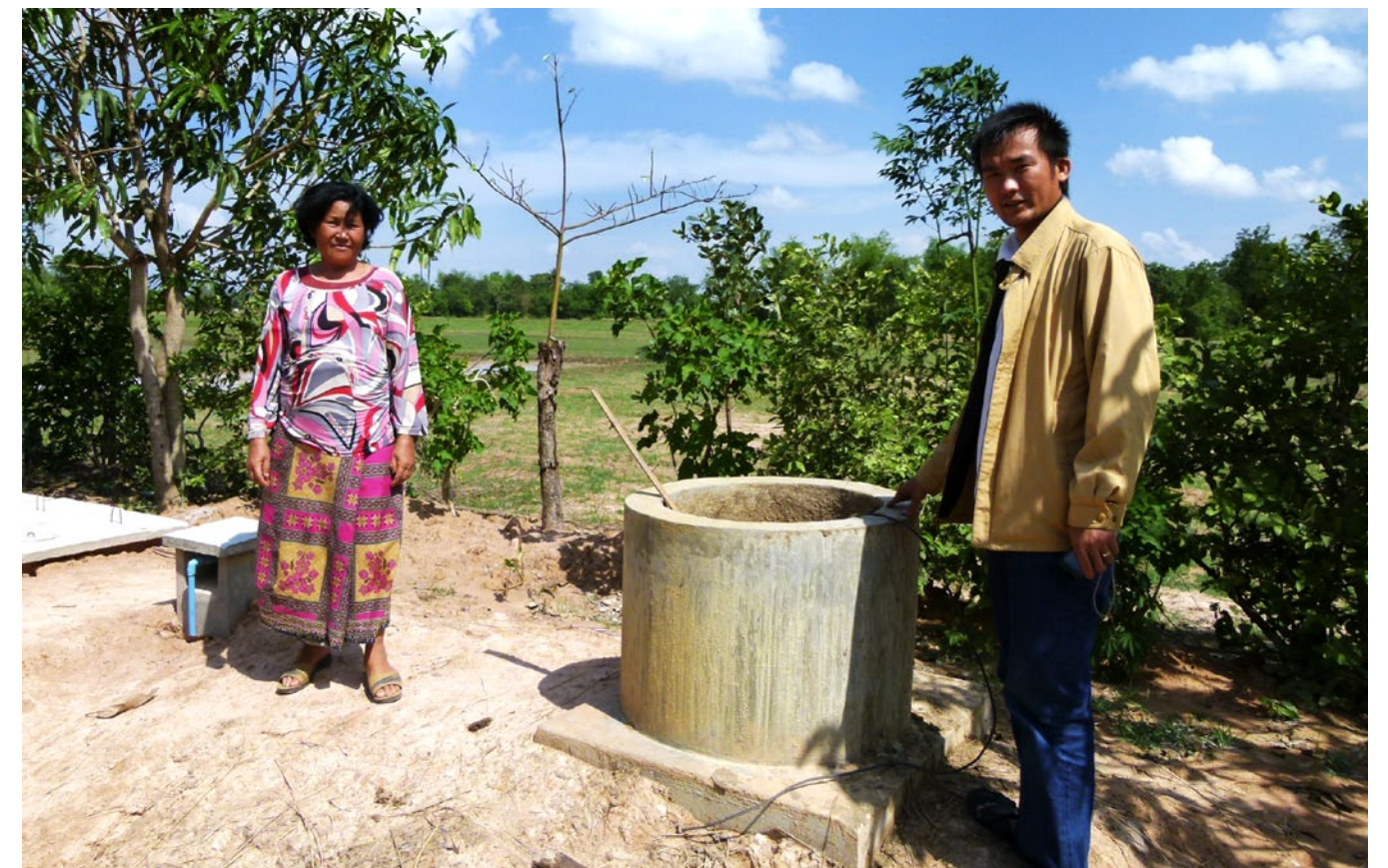
Cambodia: Construction of household biogas stations
