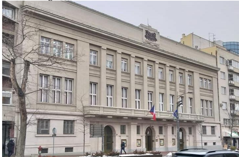
Renovation of the embassy building in Belgrade, including installation of a façade lighting system, was completed in 2022
