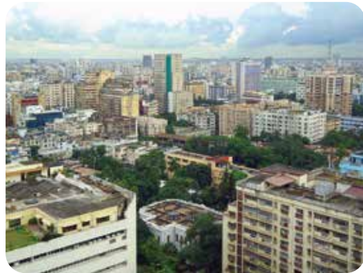
URBAN INFRASTRUCTURE & HOUSING
