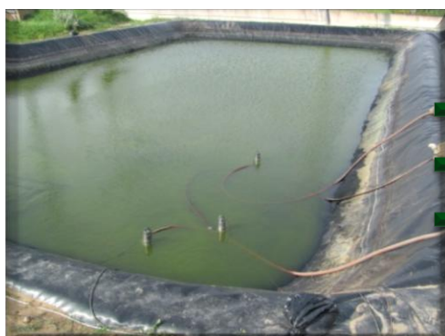
Water pumping from a reservoir to the steel tank
