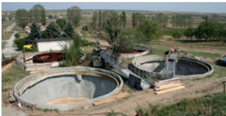
Moldova: reconstruction of a wastewater treatment system
