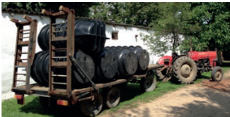
Serbia: construction of the sewage system in the Kruščica region
